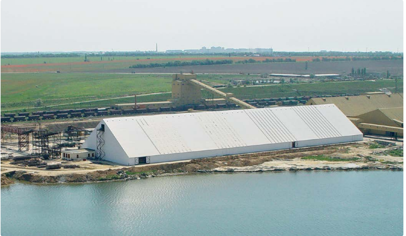
Project: TIS Port - Odessa, Ukraine | Type: PALRUF® 3mm White Opaque and Clear (Clear sheets used as skylights)
